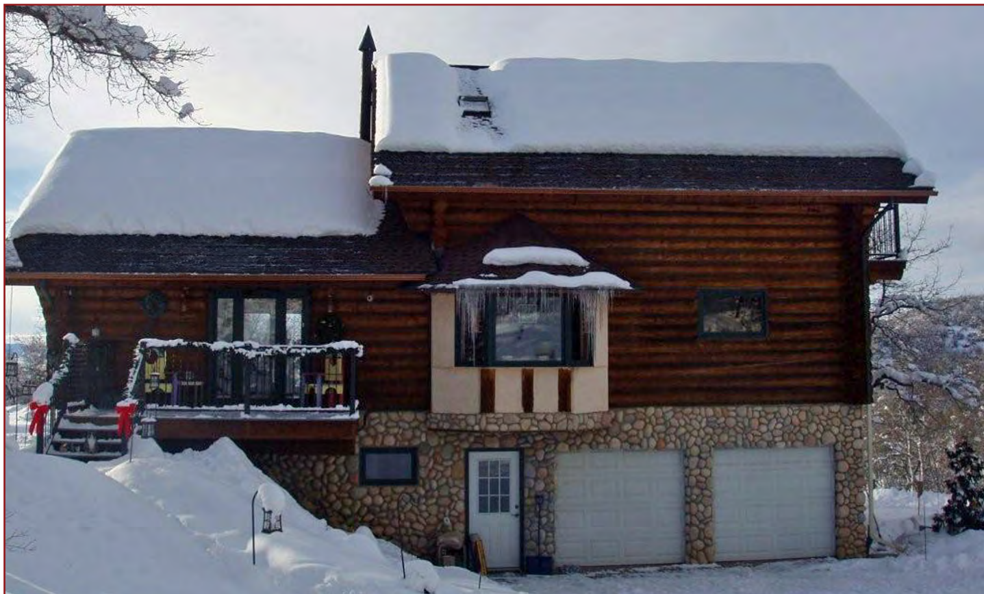
Mountain cabin with low-voltage roof de-icing system installed at the roof edges.
