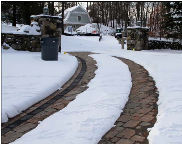
Heated paver tire track driveway
