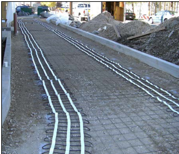
Heated tire track driveway being installed.
