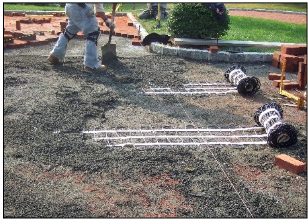
Installing ClearZone snow melting mats for heated paver driveway.
