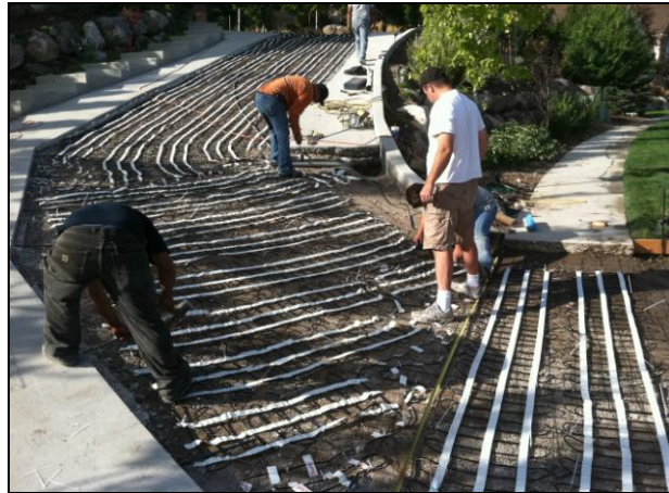
Laying out the ClearZone heating mats.
