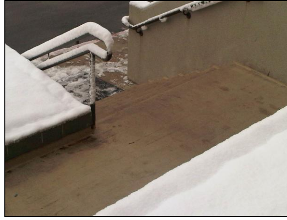
ClearZone snowmelt system installed in concrete steps.
