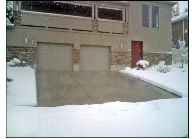
ClearZone snow melting system in operation.
