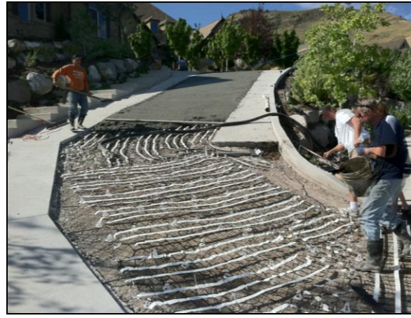
Pouring concrete over CZ heat cable and remesh.
