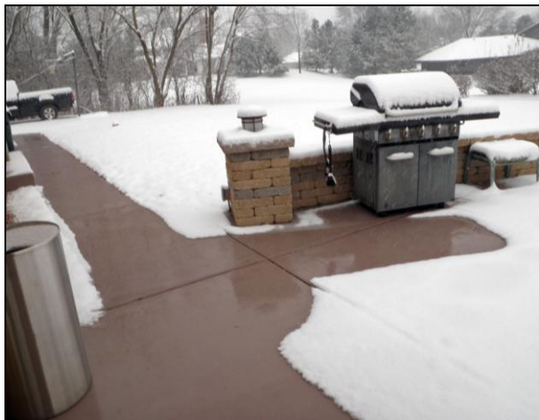
ClearZone-heated concrete patio and sidewalks.
